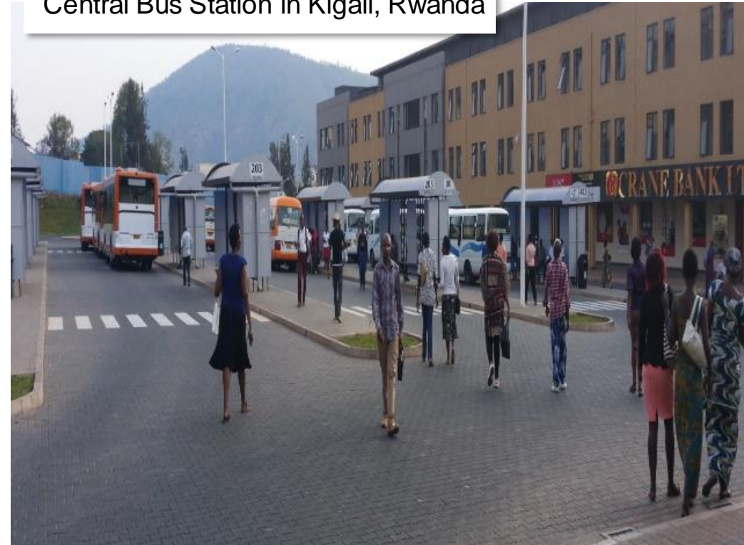
Central Bus Station in Kigali, Rwanda
